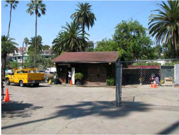
Plate 14. Park Maintenance Building (pre-1916)
