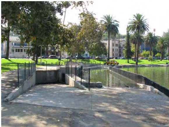
Plate 23. Stormwater Inlet Structure
