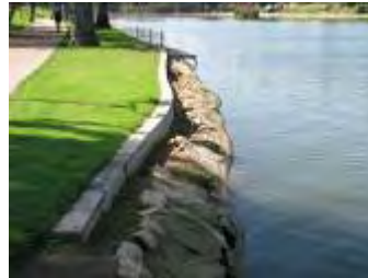
Sections of Exposed Riprap that May Survive from the 1890s
