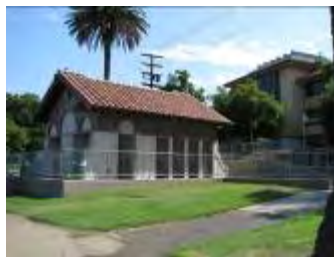
Retaining Walls Near Boathouse Restroom
