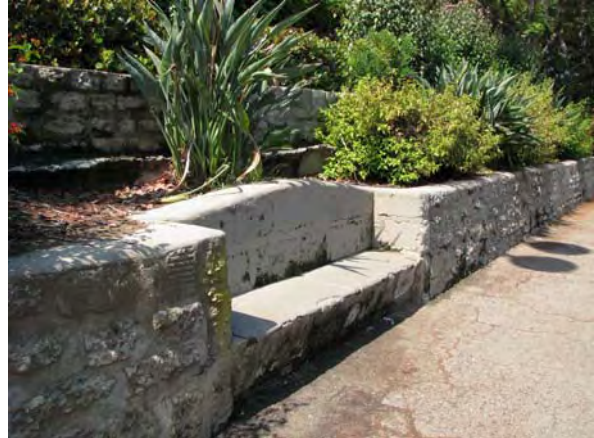
Plate 25. Masonry Retaining Walls with Three Built-in Benches
