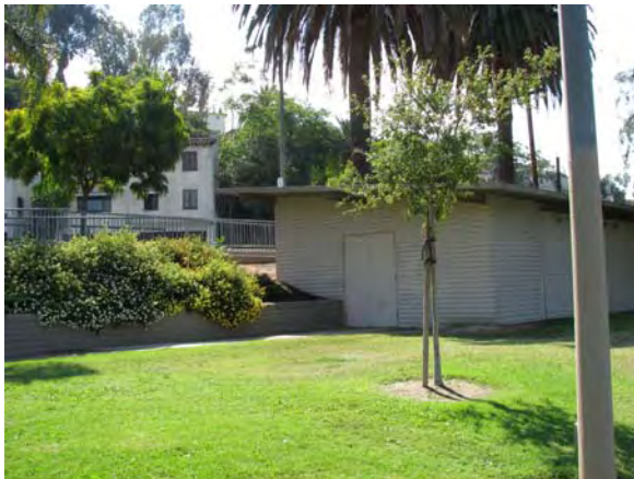
Plate 19. Concrete Block Utility Shed near Boathouse
