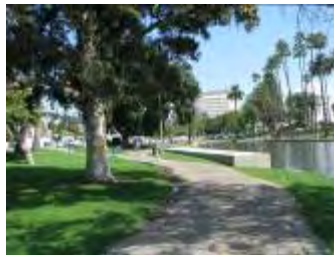
Storm Water Infrastructure Inlet
