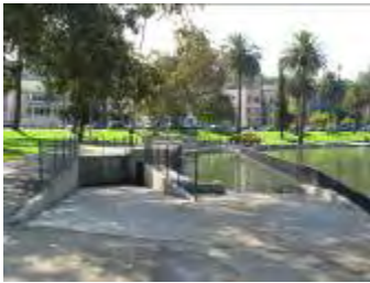
Stormwater Inlet Structure
