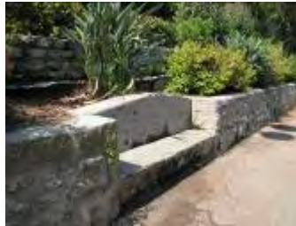
Masonry Retaining Walls with Three Built-in Benches
