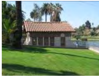
Restroom near Boathouse
