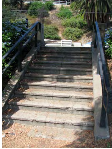
Plate 33. Concrete Steps from Street-level Pathway to Park-level Pathway (1920s-early 1930s)
