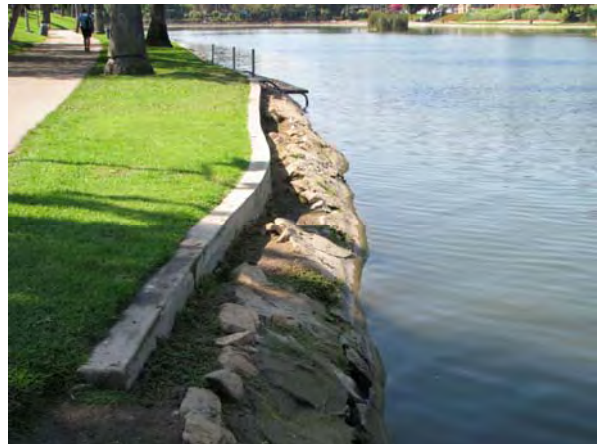
Plate 65. Sections of Exposed Riprap that May Survive from the 1890s
