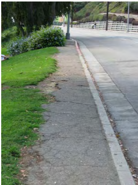
Plate 36. Sidewalks Surrounding Park (at Street Level)
