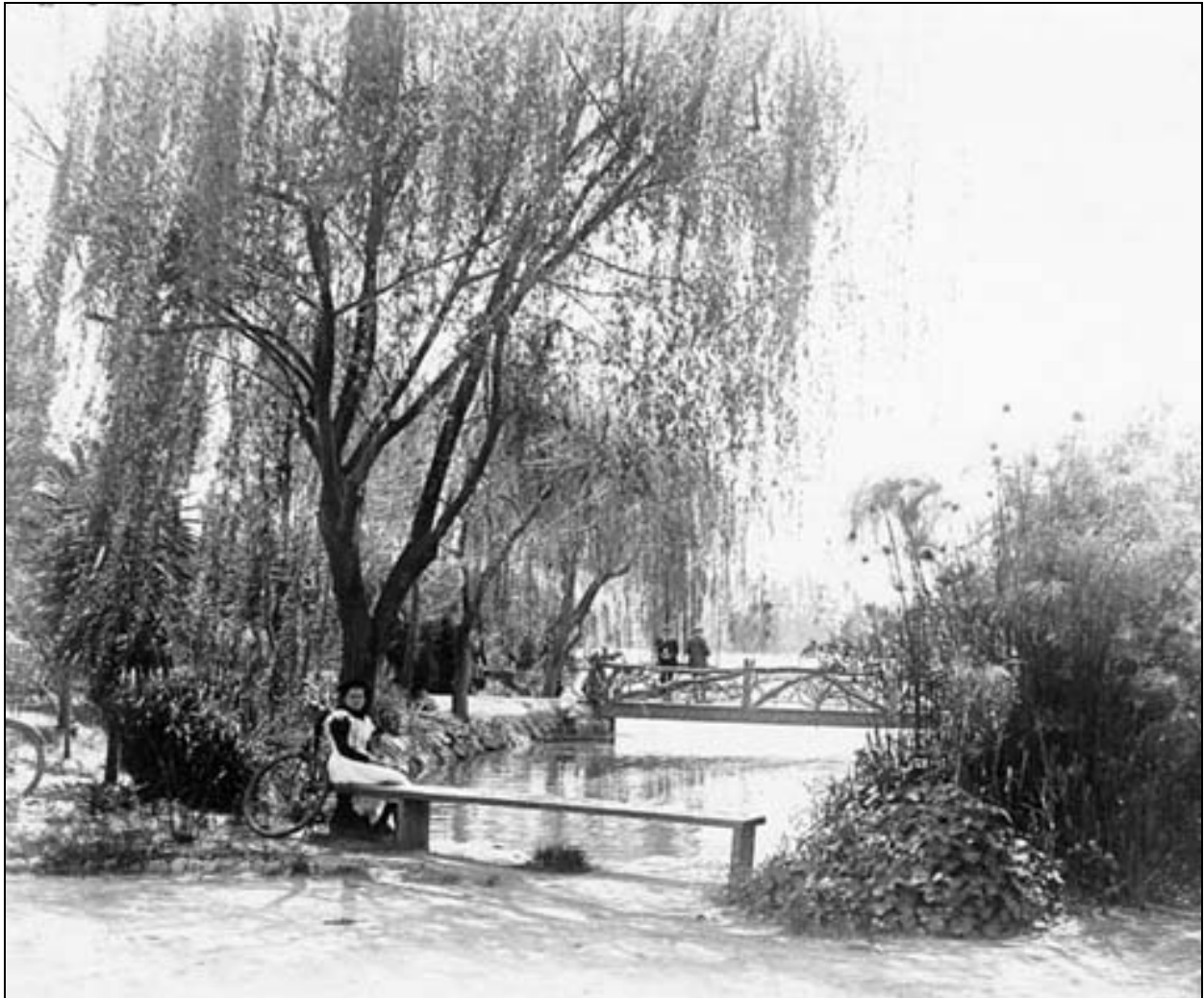
Plate 6. Flat-span Wooden Bridge in Northwestern Arm of Lake, ca. 1900 (LAPL Photo Collection).
