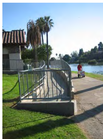
Ramps near Boathouse Restrooms
