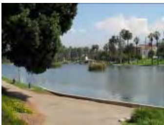
Retaining Wall/Lake Edge
