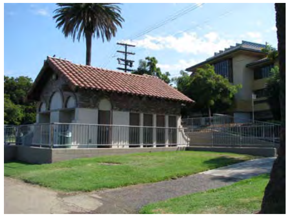
Plate 29. Retaining Walls Near Boathouse Restroom
