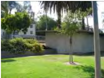
Concrete Block Utility Shed near Boathouse
